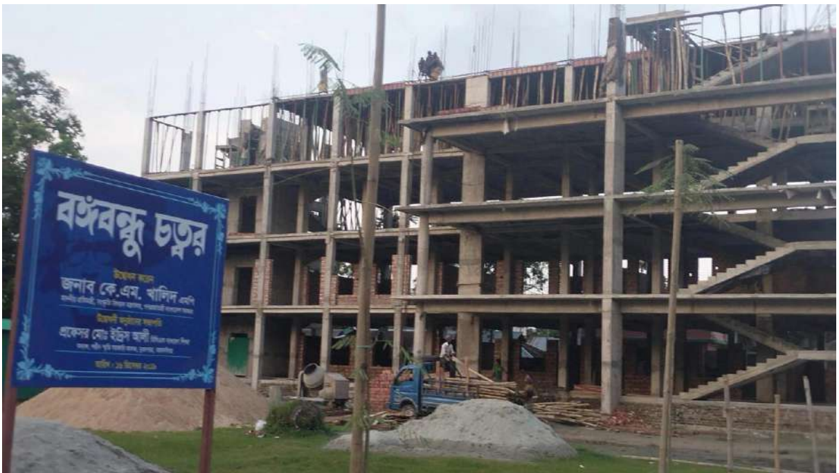
Under construction 6 Stored academic building
